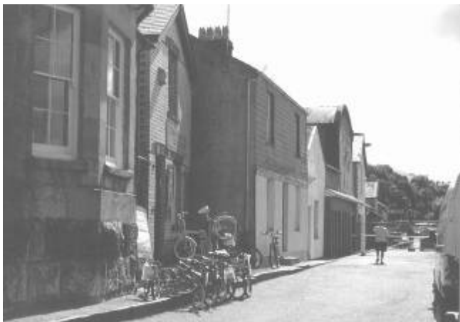
Caernarfon's Harbour Trust is seeking to demolish this entire group of buildings, industrial and residential
